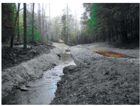
Panther Branch before restoration/Tennessee Department of Conservation
